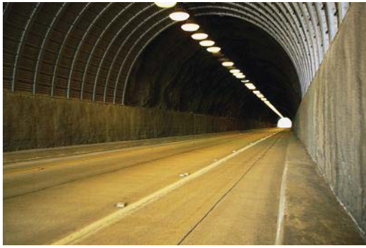
Fig. 2. Application: Tunnel Construction
